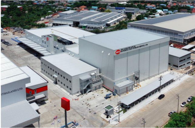
[Exterior View of the New Warehouse]
