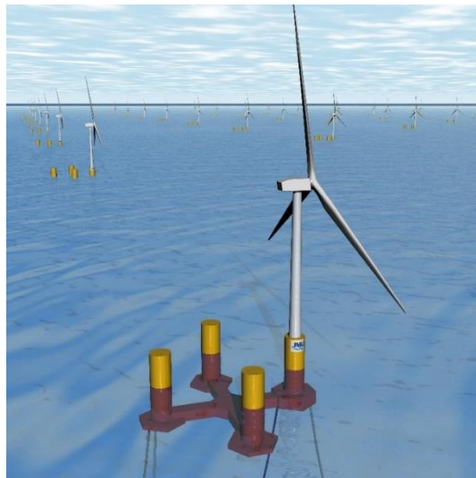
Floating Offshore Wind Turbine (Provided by Japan Marine United Corporation)
