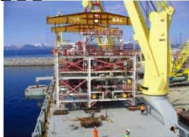
Project cargo: Assembled module of LNG plant
