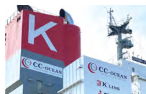
Installing CO 2 Capture Plant on vessel by CC-Ocean Project
