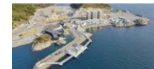
Northern Lights CO 2 receiving terminal (Under construction in Øygarden, Norway) (Image provided by Northern Lights JV DA)
