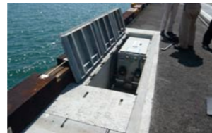
Connection box for shore power supply cables installed on the quay
