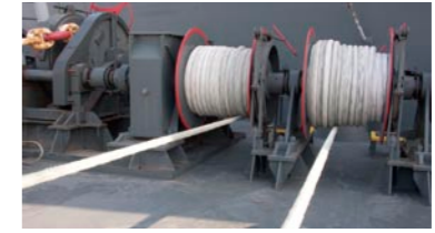
Electric mooring winch and mooring lines (forward deck)
