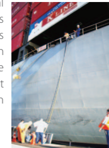
Shore electricity power being supplied to a containership
