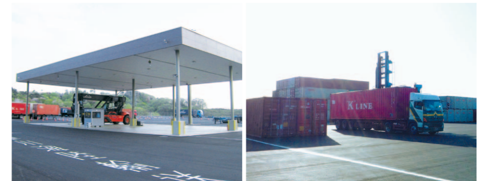
New terminal that opened in April 2013
