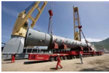
Loading operation of large reactor for oil refinery
