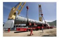
Loading operation of large reactor for oil refinery
