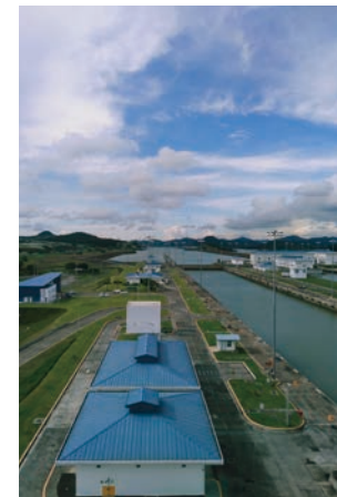
Panama Canal Neopanamax locks (to the right in the photo)
