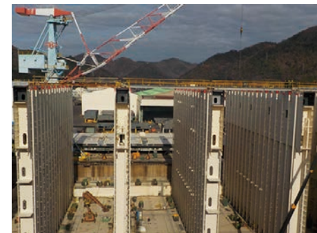
Scene of trans-bulkhead block mounting
