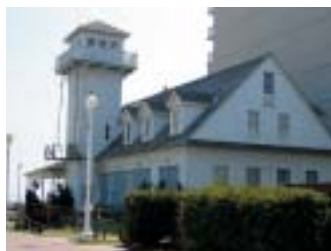
Restored Life Saving Station still stands watch over the Atlantic at VA Beach
